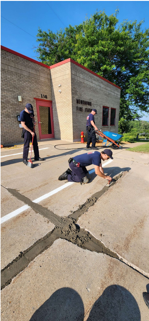
Repairing concrete
