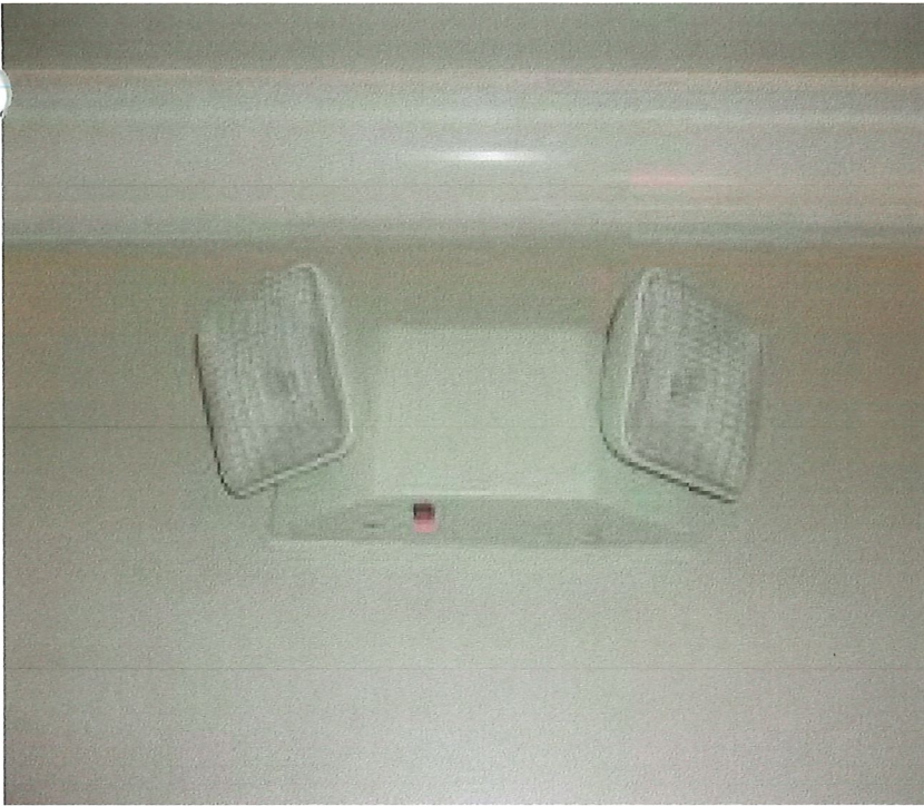
Non-functioning emergency lighting
