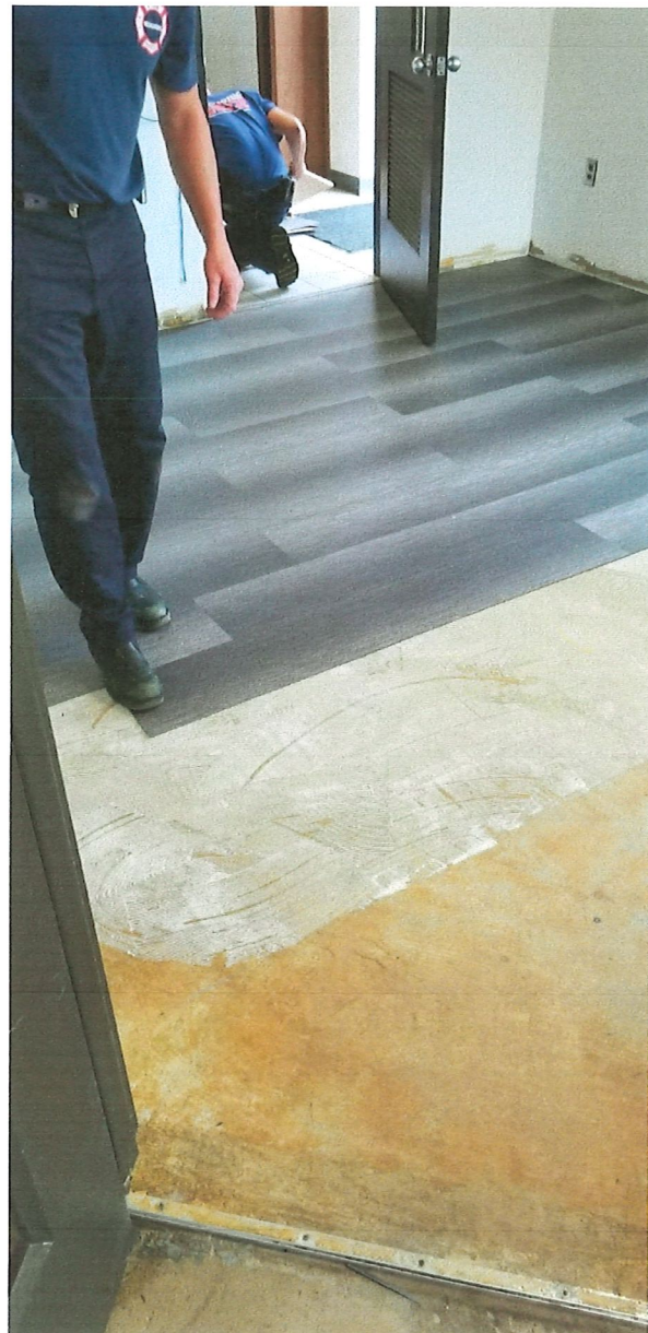
C shift at work laying flooring
